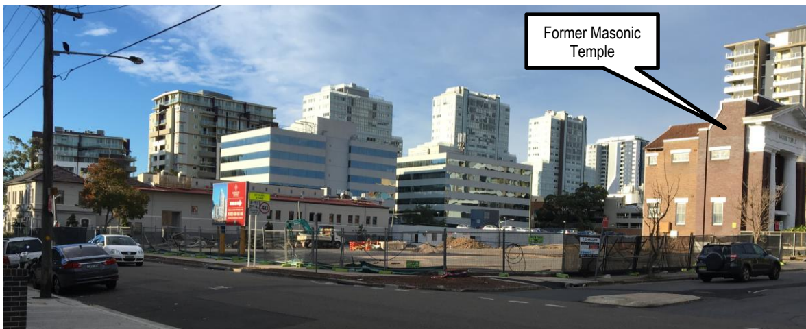
Figure 4: Western portion of the site looking north east from Conder Street
