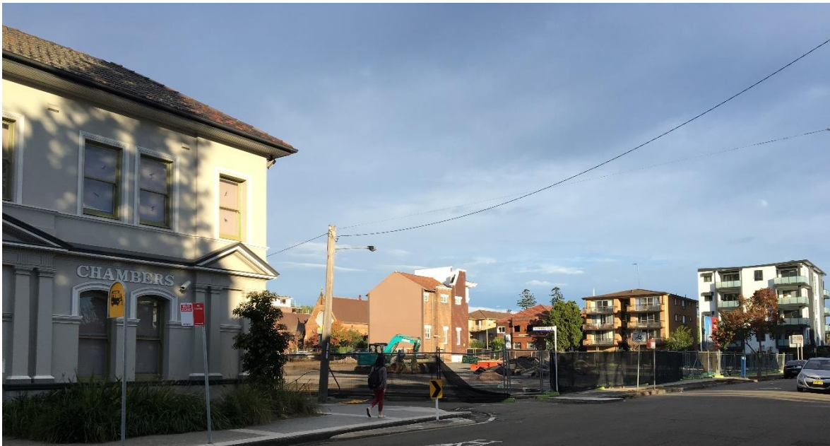
Figure 7: Hornsey Lane and Burwood library building adjacent to the north-western corner of the site
