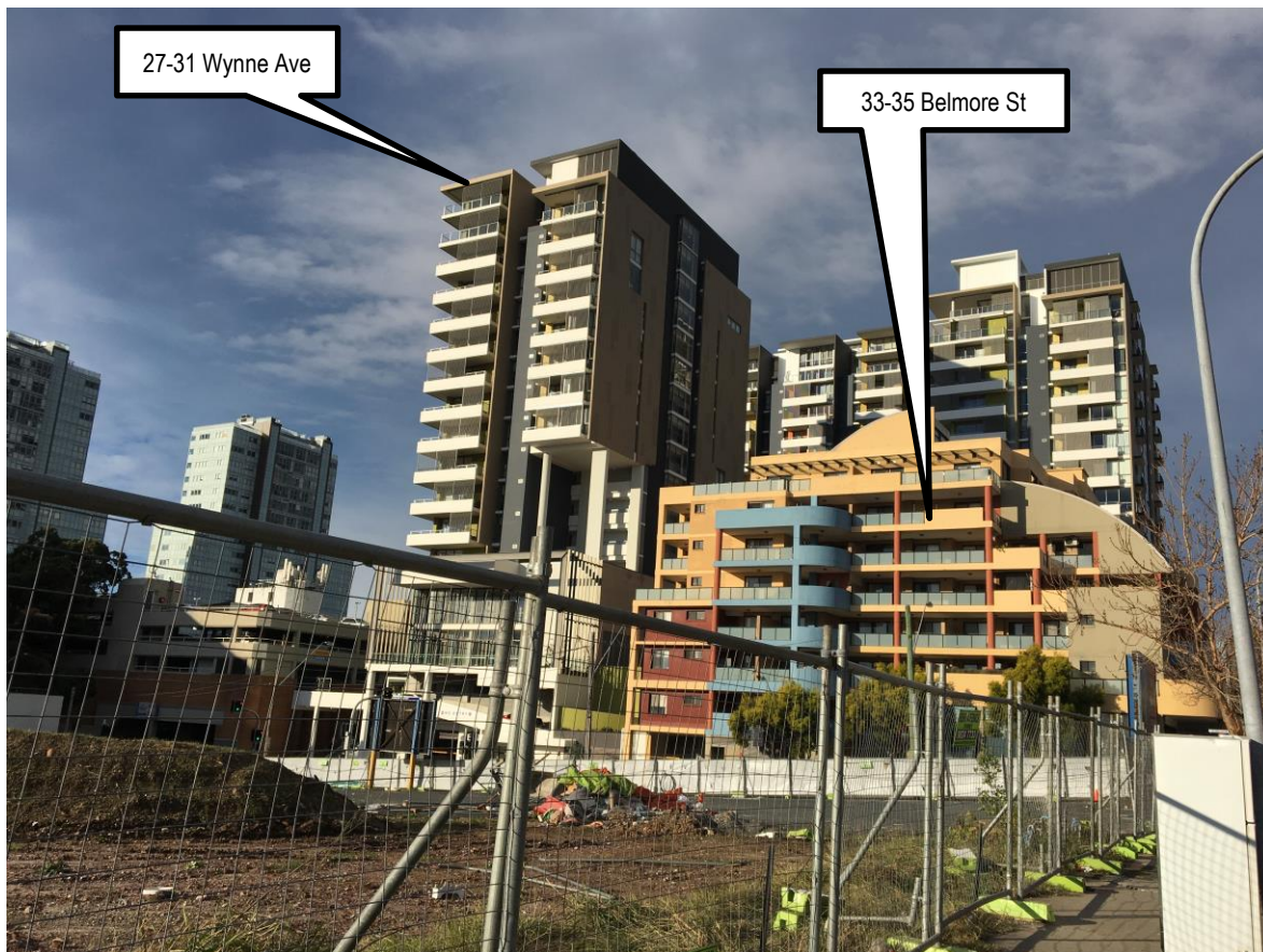
Figure 3: Eastern portion of the site looking east towards Wynne Avenue
